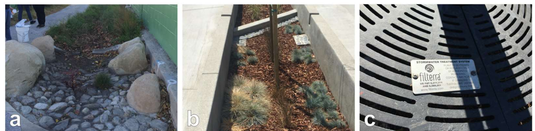
Figure 4. Examples of Los Angeles systems designed to remove debris and contaminants from runoff: (a) biofilter along Elmer Avenue Paseo, (b) biofilter in the Avalon Green Alley, and (c) Filterra™ bioretention system on Grand Boulevard.
